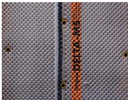
Delta Qwik-Seal Plug installed into the waterproof membrane
