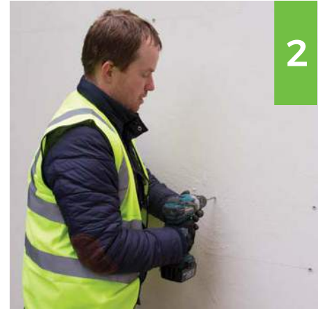
Drill the holes
