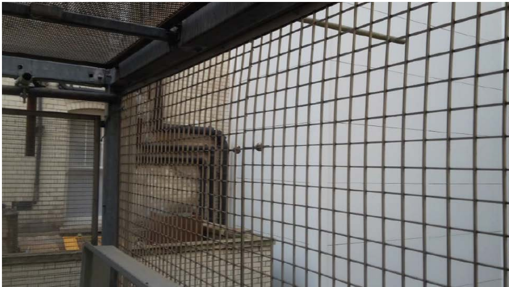
Metal cage before Vistafolia ® installation
